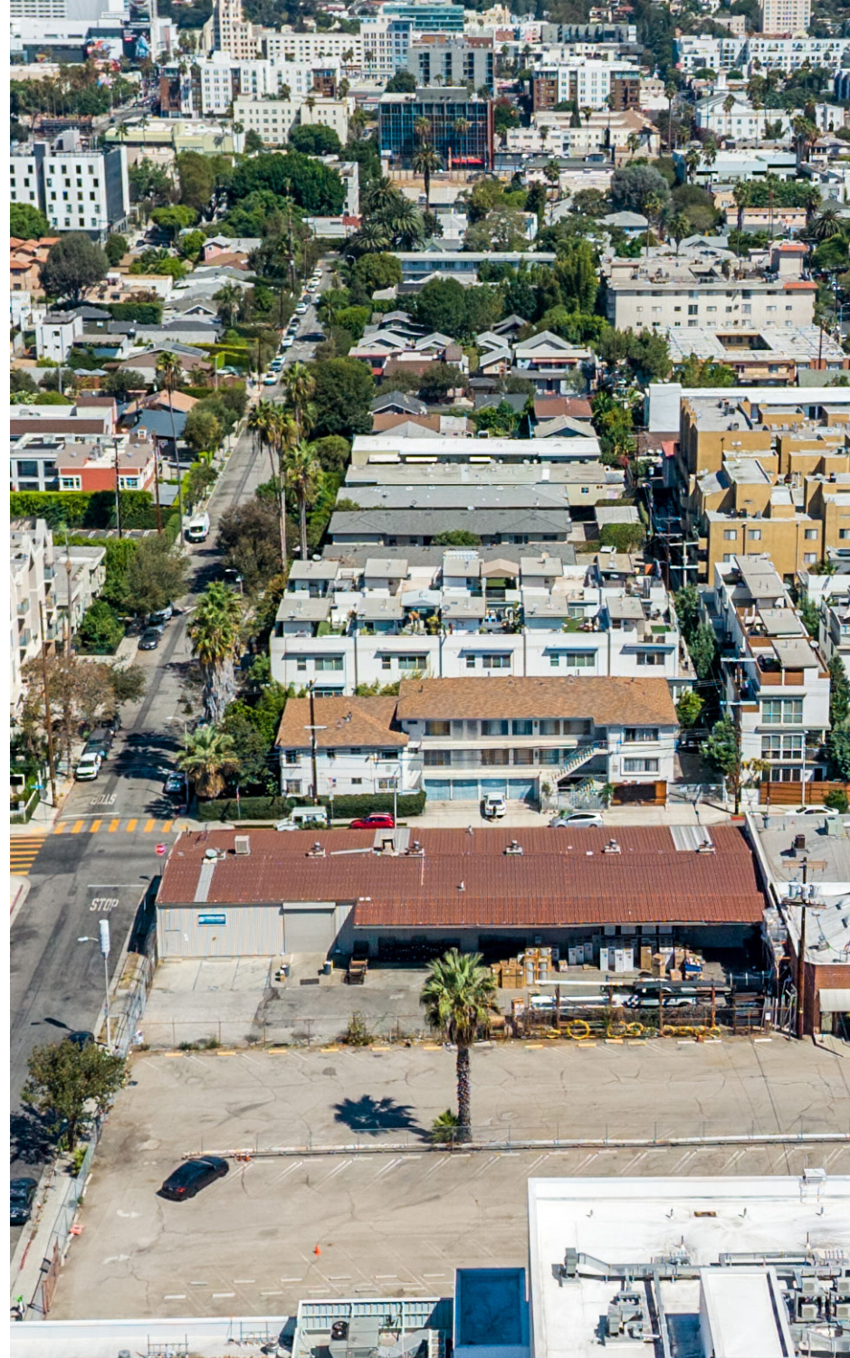
BUILDING AND YARD · FROM THE NORTHWEST
