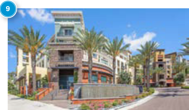
The Boulevard Apartment Homes 20600 Ventura Blvd
